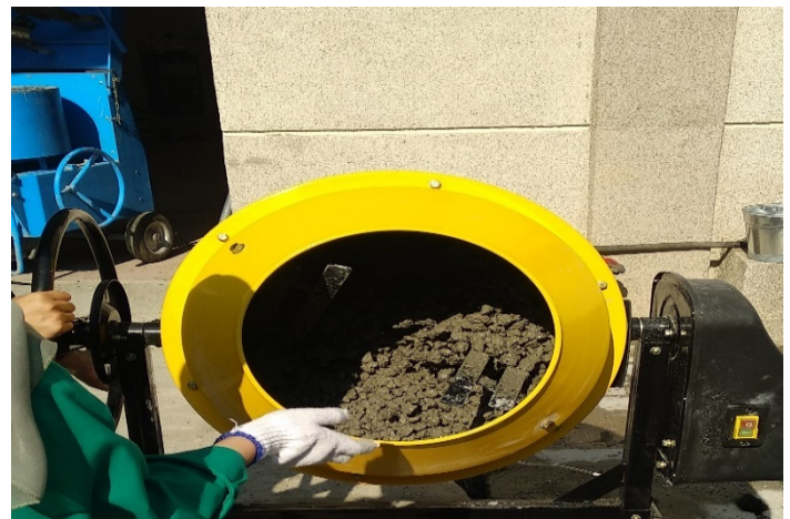
Figure 4: Concrete mixing by using concrete mixture machine
