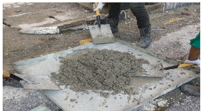
Figure 5: Concrete mixing by hand mix
