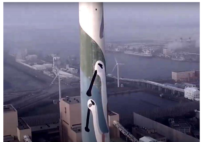
Figure 10: Chimney painted with images of animals [14].
