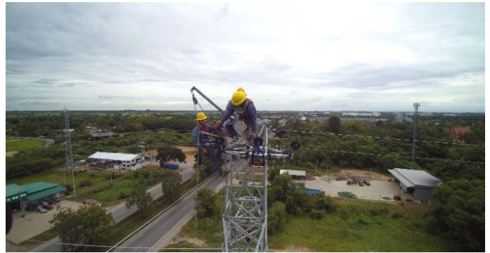
Figure 20: Actual field test on a 115 kV transmission line
