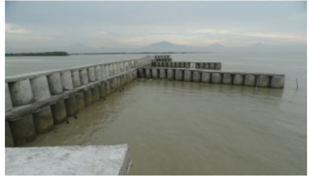
Figure 5: Breakwater of concrete buis type built on 2012.
