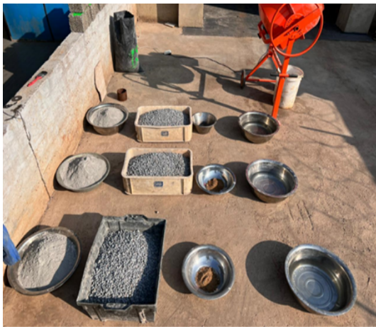
Figure 8: Weighed and sorted material according to the mix design.
