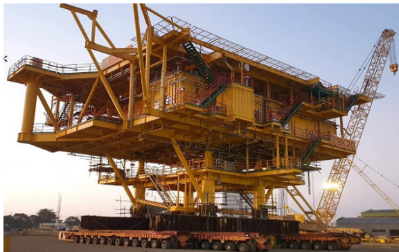
Figure 1: A project to load out the gantry using self-propelled trailers
