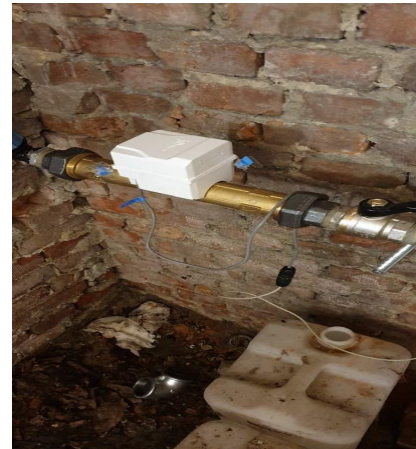
Figure 6: Installation of the meter water in the school
