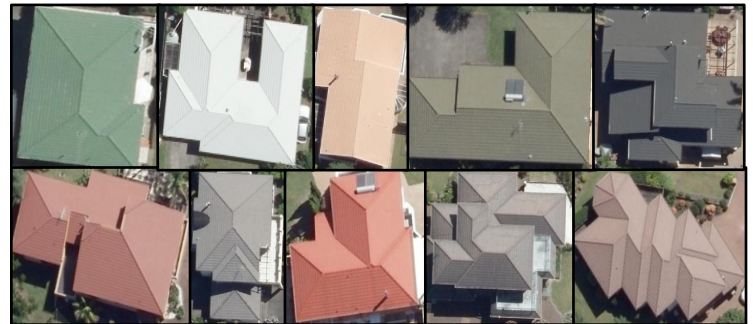
Figure 2: Aerial images of buildings in the study area New Zealand from various perspectives
