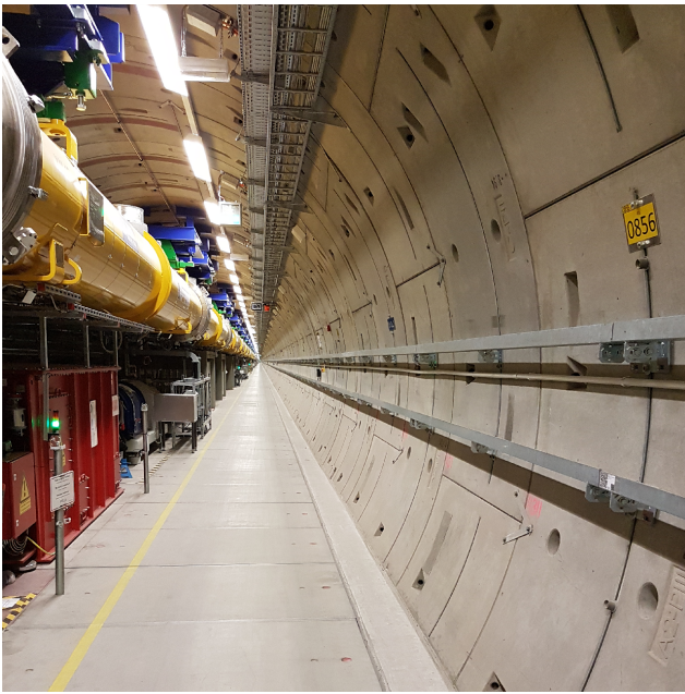
Figure 3: View along the XFEL tunnel
