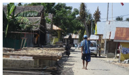
Figure 9: Condition of roads (Source: Authors, 2018)
