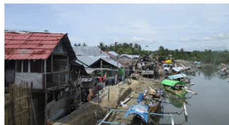
Figure 8: Houses with mooring (Source: Authors, 2018)
