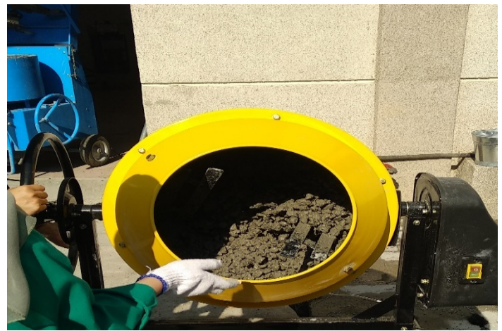
Figure 4: Concrete mixing by using concrete mixture machine
