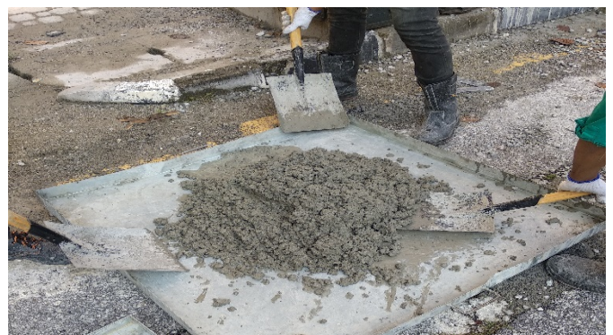
Figure 5: Concrete mixing by hand mix
