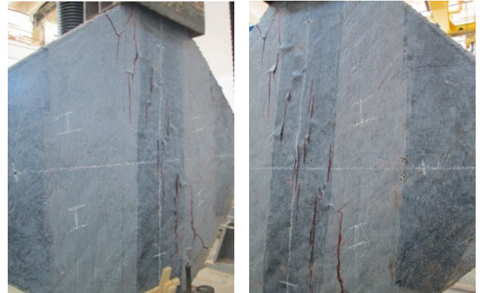
(a) Delamination and shear cracking (Side I)
