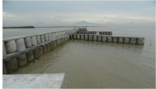
Figure 5: Breakwater of concrete buis type built on 2012.
